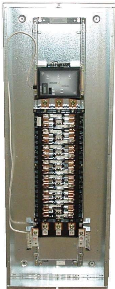
Integral TVSS with Long Neutral Conductor
