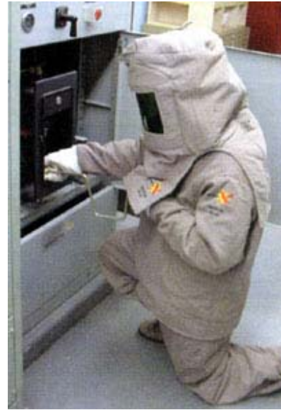
FIGURE 3 ARC FLASH & PPE
